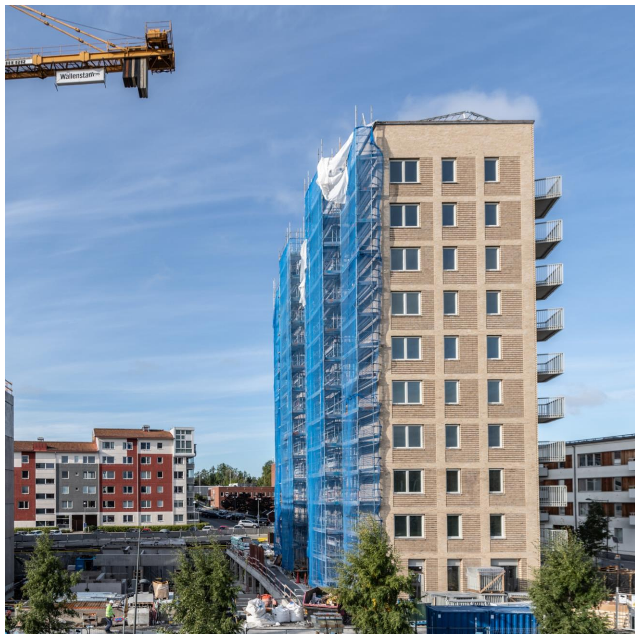
Terrassen Elva & Allén, Tyresö – 275 lgh
