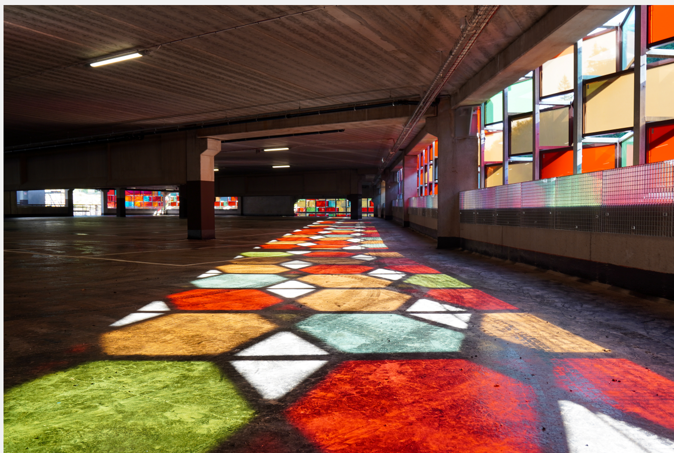
Garage facade with PV plants - Mölnlycke
