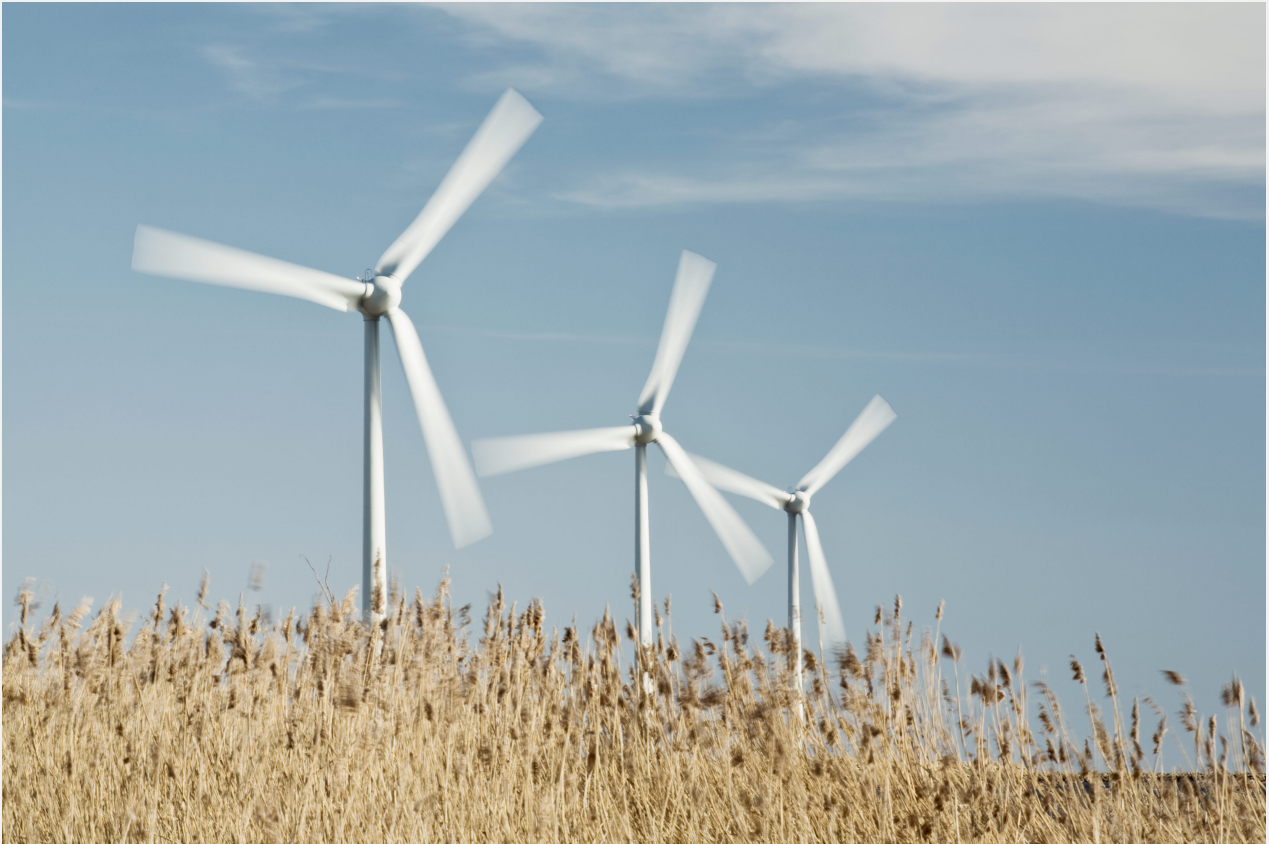
Kilagården wind farm - Skara
